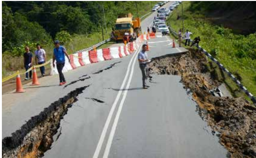
Jalan rosak akibat tanah runtuh di sepanjang Jalan Pan Borneo, Bukit Song, Lambir, Miri, Sarawak Road damaged due to landslide along the Pan Borneo trunk Road, at Bukit Song, Lambir, Miri, Sarawak.
