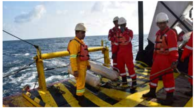
Sonar imbasan sisi dan boomer sedang diturunkan bagi melaksanakan survei geofizik Projek Kajian Sumber Pasir Laut Negara Fasa 3 – Lepas Pantai Pahang dan Johor Timur Deploying of side scan sonar and boomer for geophysical survey of National Offshore Sand Resource Study Phase 3 – Offshore Pahang and East Johore
