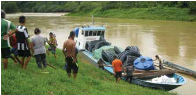
Penghantaran paip, tangki dan kelengkapan lain untuk Sistem Air Graviti Bukit ke Rh Belikau, Bahagian Kapit, Sarawak Delivering of pipes, tanks and accessories for the construction of a gravity-fed water system at Rh Belikau, Kapit Division, Sarawak
