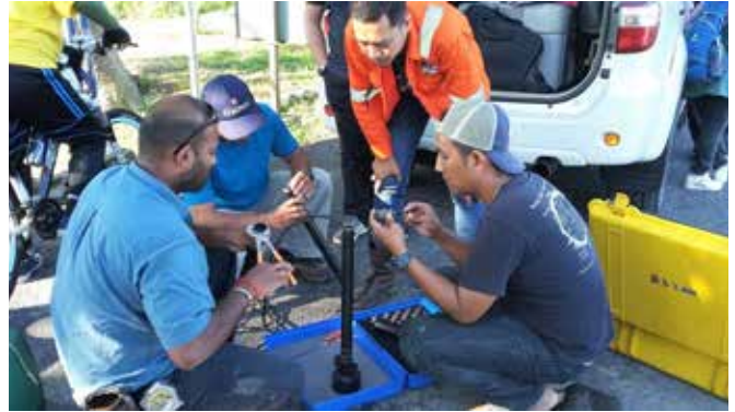
Pemasangan echo sounder Installation of echo sounder
