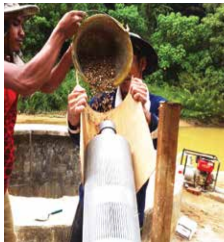
Penyediaan paip UPVC berskrin dua lapis di Raub, Pahang Two layers screen UPVC pipe preparation in Raub Pahang
